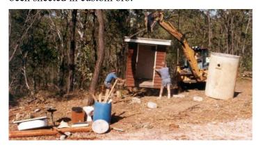
The toilet block, along with a septic system was built around a no longer used **Lakes Creek Railway Station** and a steel tank stand was constructed beside it. Having a 15,000 litre poly tank on top of the stand worked out well but because it was not engineered, it couldn't be looked upon as safe.
