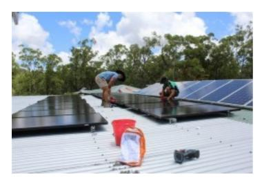
The new Solar power system includes a more up to date battery storage system and later around March a new Diesel generator will replace the old 17KVA Petrol model
